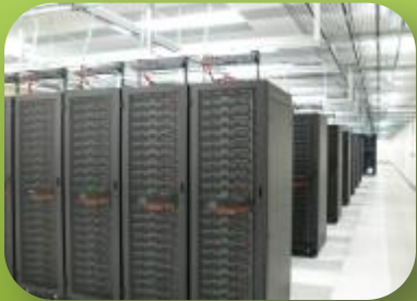
Datacenter Colocation Generation 1
