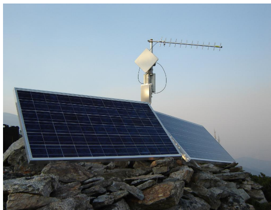
Figure 5: The Backhaul link set up on Boulder Peak. To the near side is an Access5830 with a directional antenna. On the far side is a M900S connected to a Yagi antenna. Below are two of the solar panels we used to provide power.
