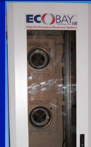
Sanmina-sci ecobay (25KW)
